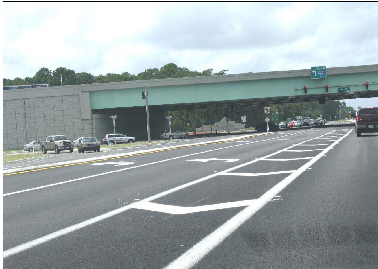
SR 100 westbound at Interstate 95 Interchange
