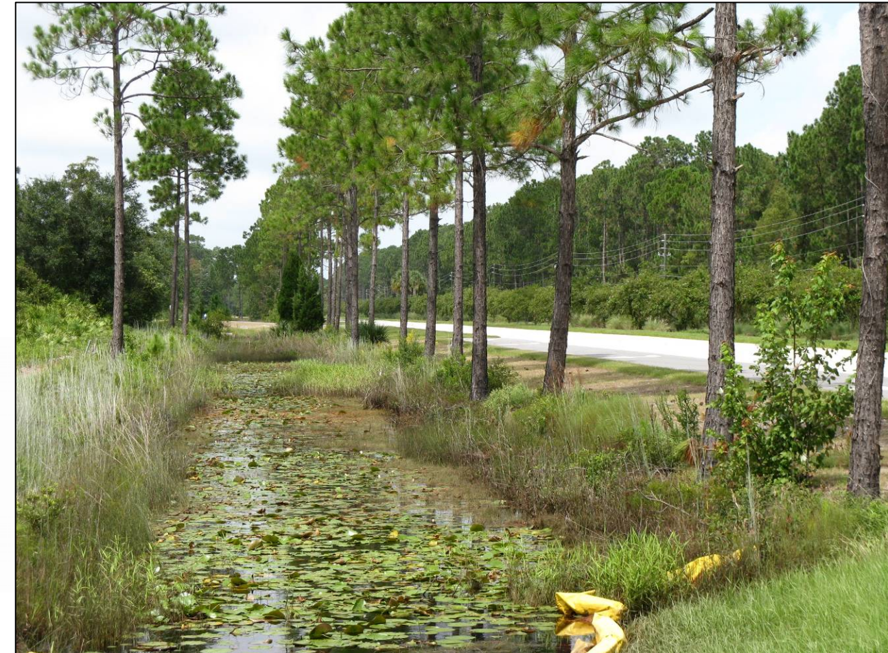
Drainage Facility along Seminole Woods Parkway
