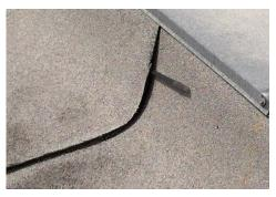
Membrane flashing problems represent the most common example of roof failure. The flashings in this area have failed, and patching is a temporary solution at best. We propose to remove the loose and deteriorated flashings and install the Self Flashing Flexbond Roofing System to eliminate such problems.
