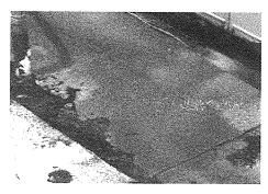
Some of the HVAC units do not have condensation lines with some leaking from the pan. Consequently there is water constantly on the roof which leaches the oils from the roof and can allow the plants to grow and deteriorate the roof. We propose installing the condensation lines and repairing any damage to the roof.
