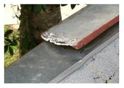
The metal cap is failing, pulling loose in places or not retaining contact to the wall in others. We propose to use raised metal drip-edge on three sides to direct all water flow to the gutter.
