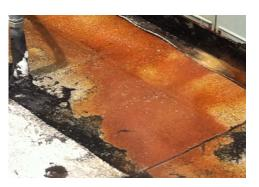
Some of the HVAC units do not have condensation lines with some leaking from the pan. Consequently there is water constantly on the roof which leaches the oils from the roof and can allow the plants to grow and deteriorate the roof. We propose installing the condensation lines and repairing any damage to the roof.
