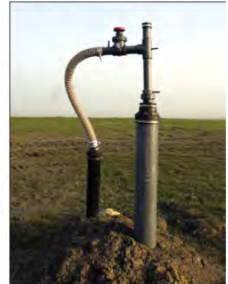
Gas extraction wells like this one collect landfill gas for destruction in a flare.
