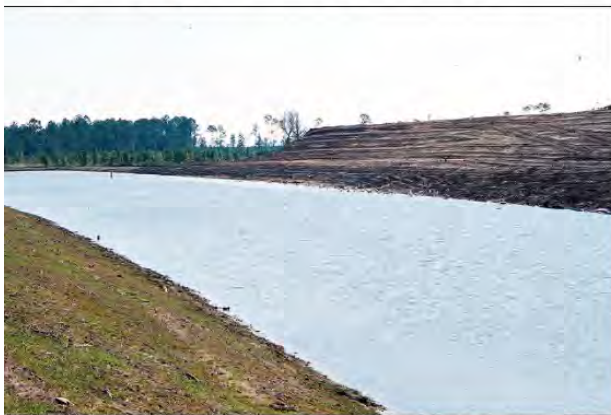
This storm water retention pond at Chesser Island Road Landfill was constructed to collect and control surface water runoff from the landfill.
