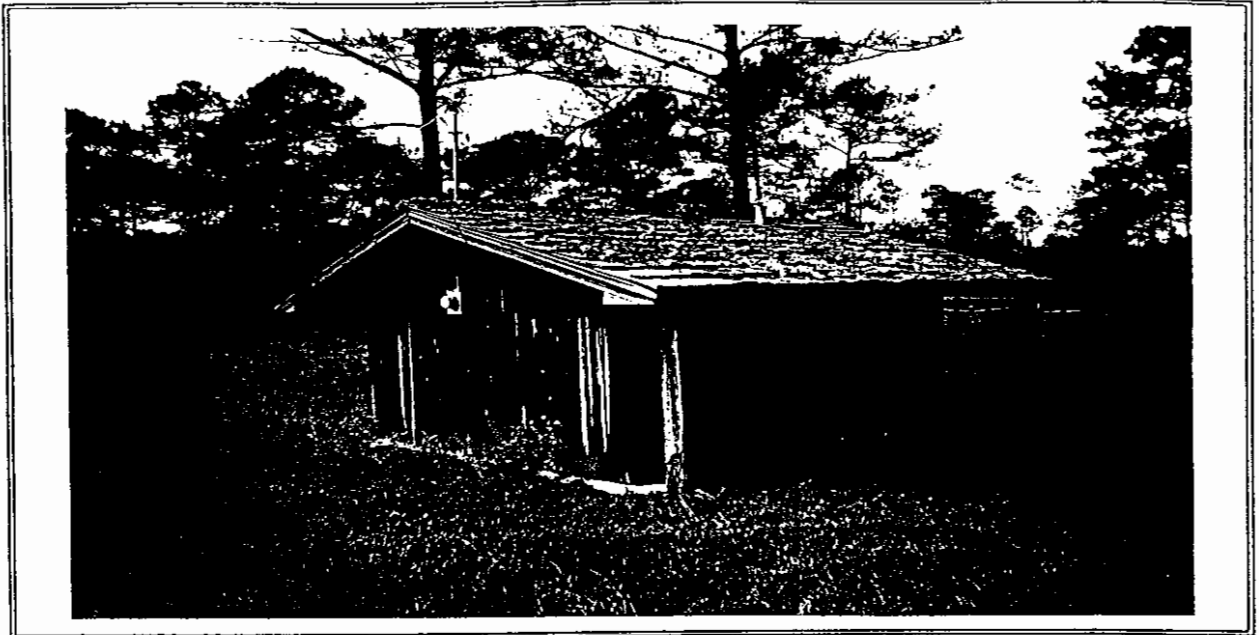
7. VIEW OF THE PUMPHOUSE ON PARCEL B
