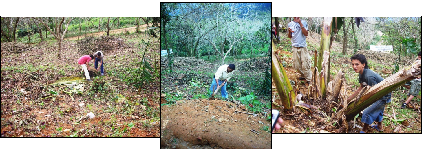
Clearing the Land!
