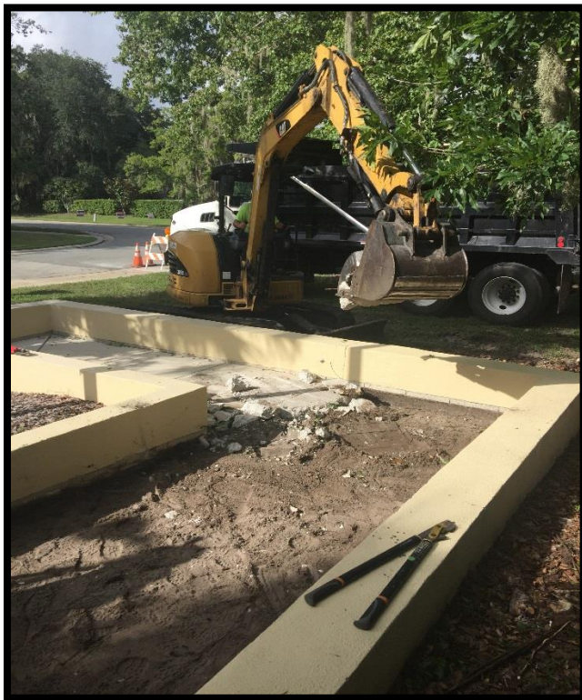
Sidewalk Installation @ Fire Station 22
